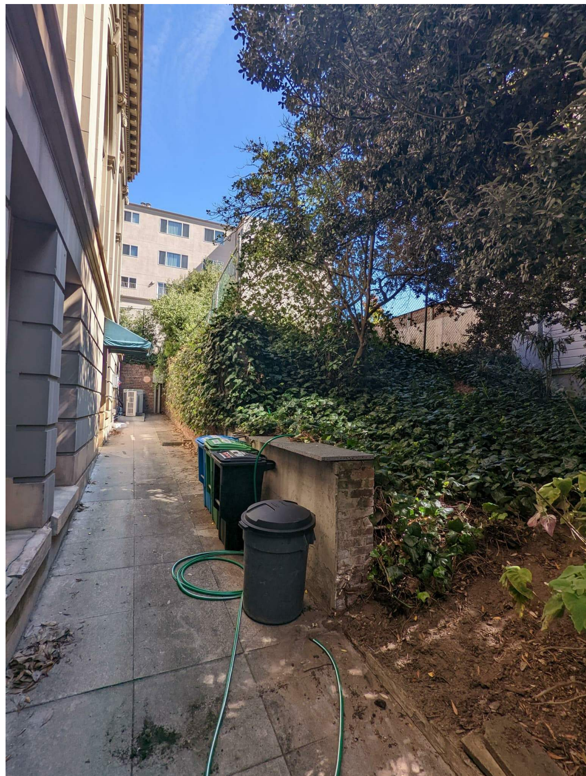
9. LOOKING AT SOUTH FACADE AT GRADE
